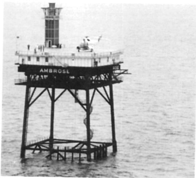
The Ambrose Offshore Light Tower, 7 miles east of Sandy Hook, New Jersey. Its primary light has a high intensity of 6 million candlepower with a charted range of 18 miles.
